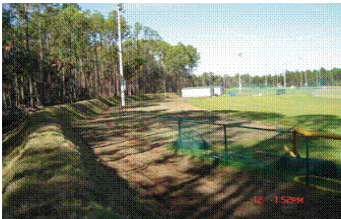
MER’s team constructs 800’ containment berm .
